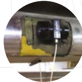
Modern technical fabrics make it possible to produce special versions of the SUM Chemical Guard covers that signal gasket rupture through a color change in the exterior cladding - the perfect solution for insulating flange connections.
