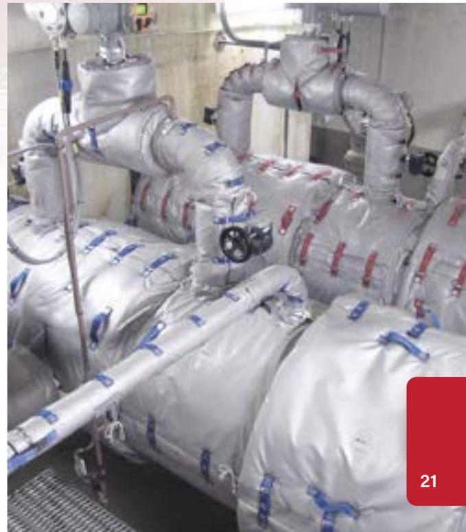
■ The technology of thermal insulation covers is now widely recommended by practically all turboset manufacturers.
