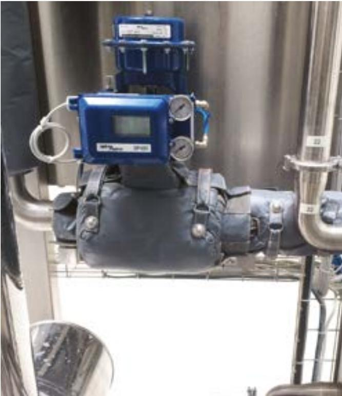
Thanks to the use of special insulating materials, **SUM Higienic Guard®** is widely used on ammonia, glycol or ice water installations. They eliminate the problem of sublimation or the growth of ice encasement often found on exposed parts of cooling installations. They significantly reduce the time of possible service actions and increase the energy efficiency of transmission lines.
